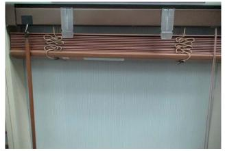
**2.** Remove the blind from the mounting brackets.
