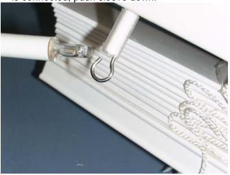
**15.** Turn wand to ensure the slats tilt correctly.
